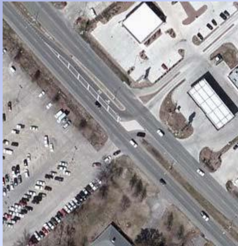
Isolated Directional Median Opening US 61 between E. Cornerview St. and Roddy Rd. in Gonzales, LA
