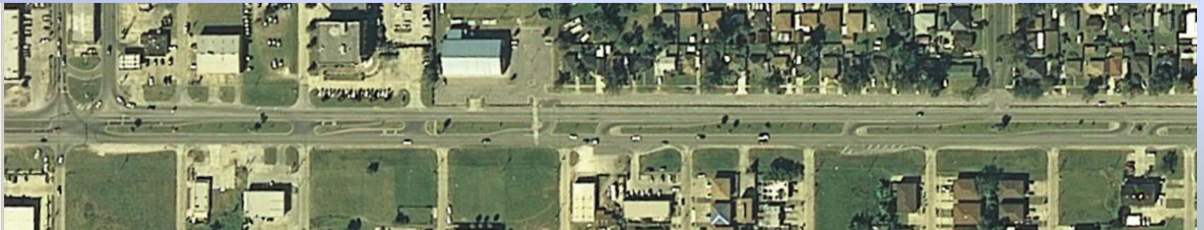
Veterans Memorial Highway in Kenner, LA (Constructed in 2005)
